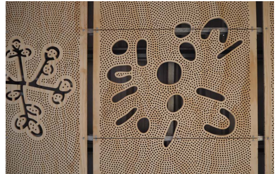
High ceilings allow for ventilation. Perforated plywood panels line existing Art Centre verandah.
