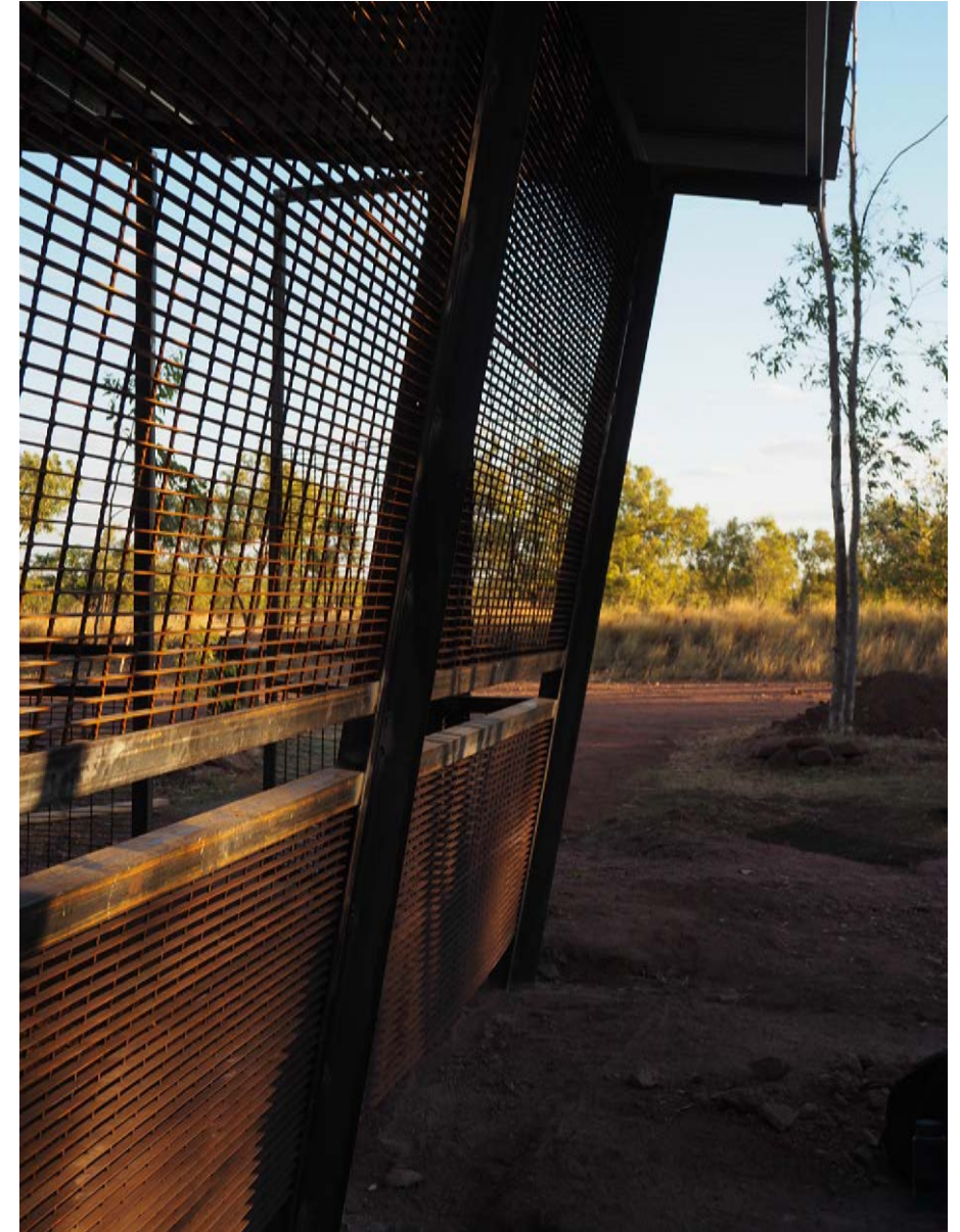
A datum line and break in the weldmesh cladding enables clear views out of pavilion when seated inside.
