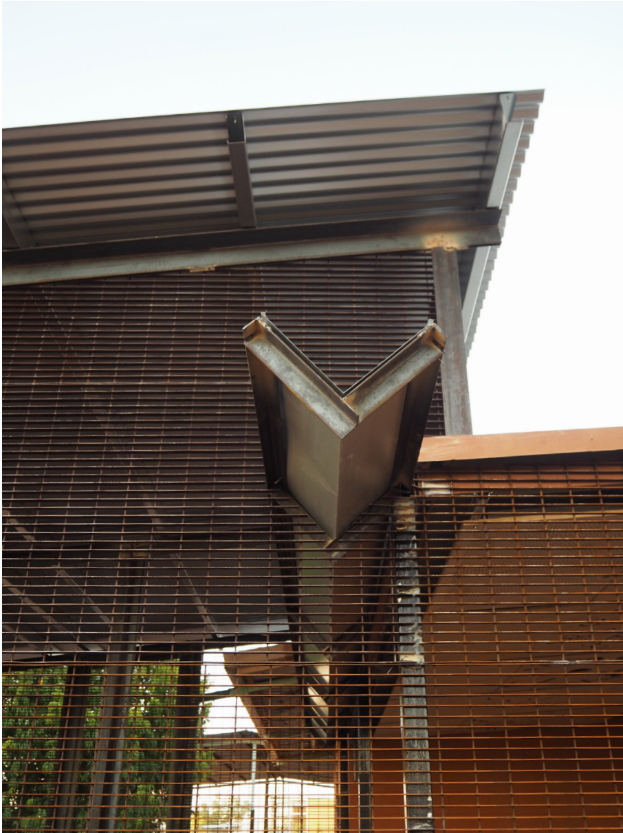
40 New gutter installed at junction between existing and new shade structures.
