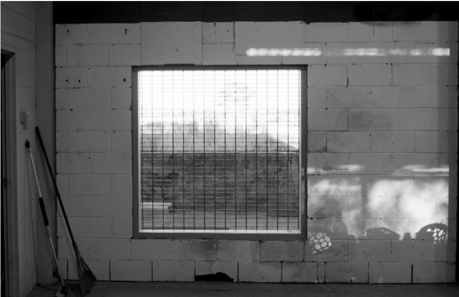
New windows recovered old openings in the building, providing much needed cross ventilation
