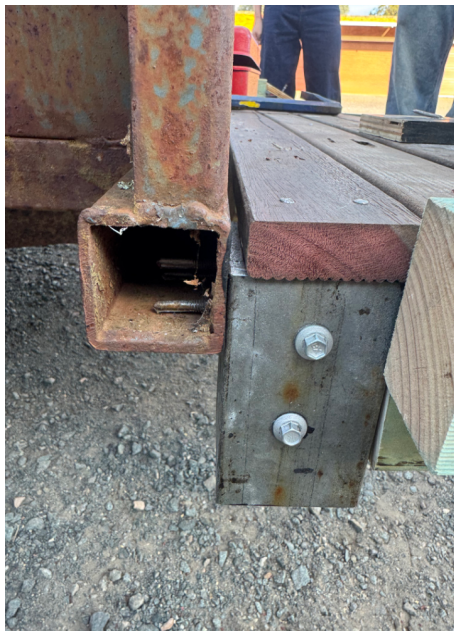
Figure 1.4 Checked in joint decking.
