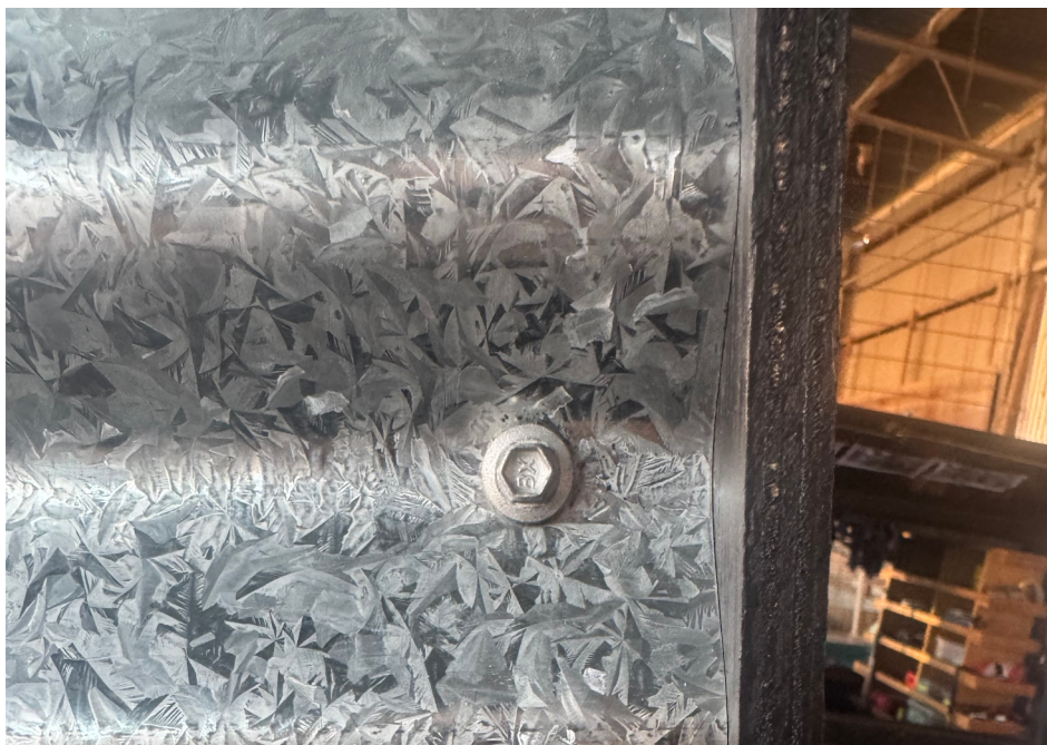
Figure 1.8 Corrugated and Ply intersection.
