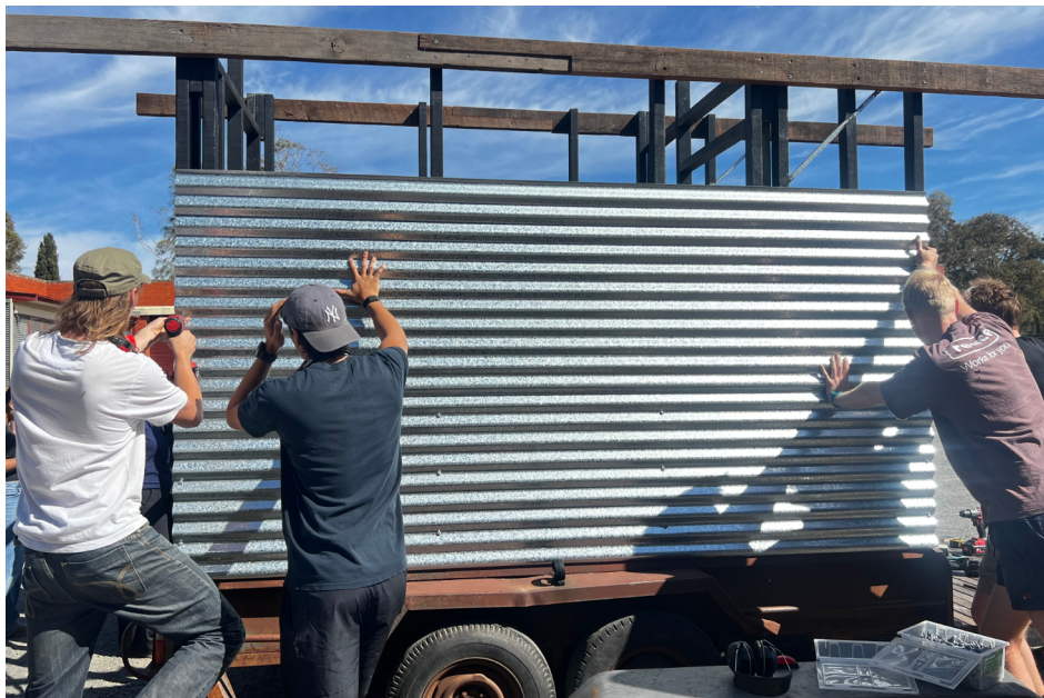
Figure 1.7 External Cladding being fixed into place
