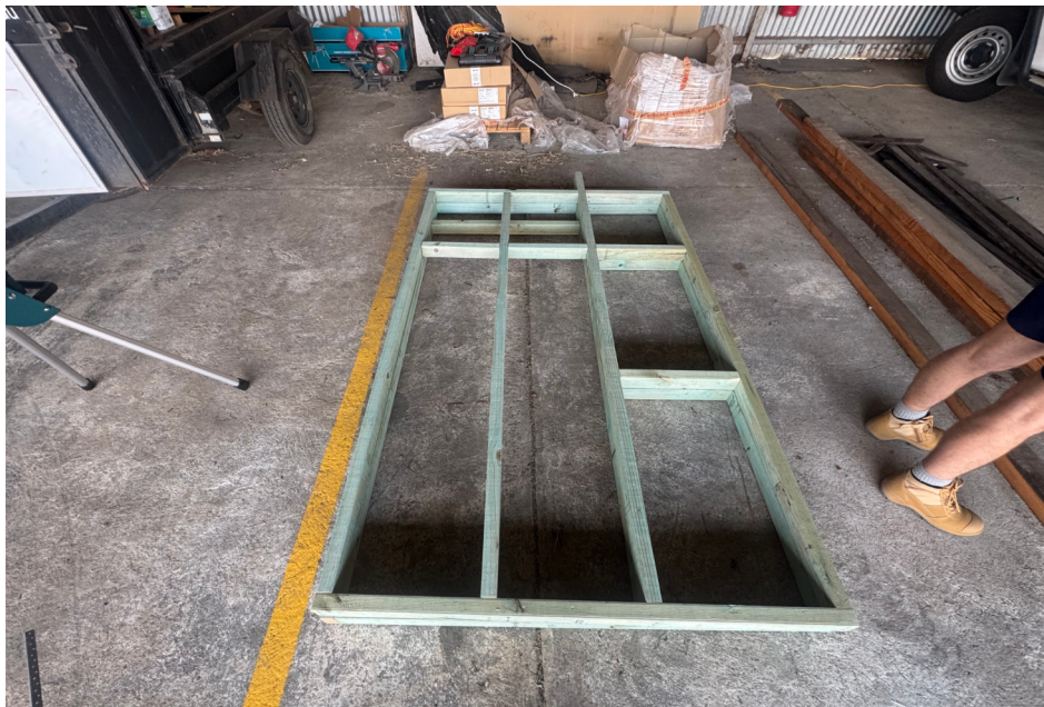
Figure 1.2 Back wall frame.
